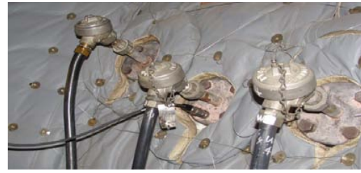
(a) Vibration measurement on the operating gas turbine
